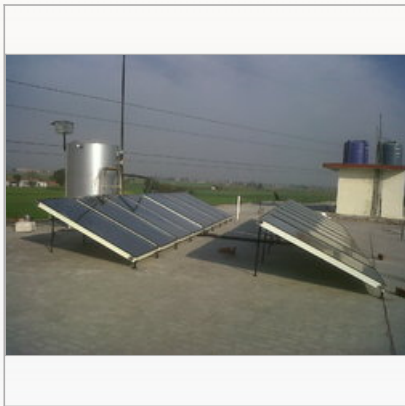
Solar Water Heater FPC With Heat Exchanger
