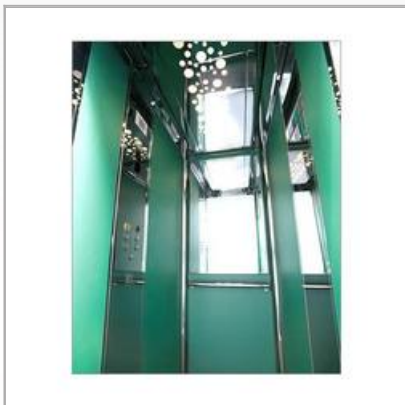
Passenger Lift And Capsual Lift
