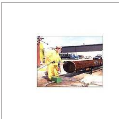
Heat Exchanger Con. Evaporator Tube - Pipe Cleaning
