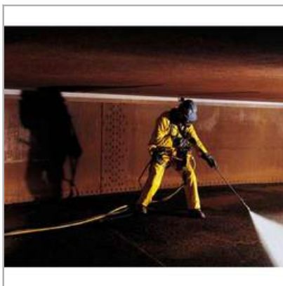
Storage Tank Cleaning Equipments
